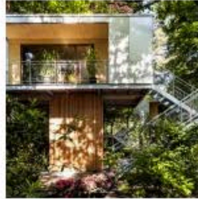
Urban Treehouse in Berlin Zehlendorf, Germany by Baumraum
