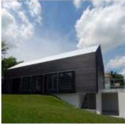
Prescott Passivhaus in Kansas City by Studio 804
